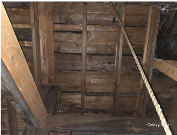
An area of the church attic before project
