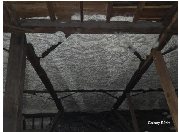
Portion of the church attic with insulation
