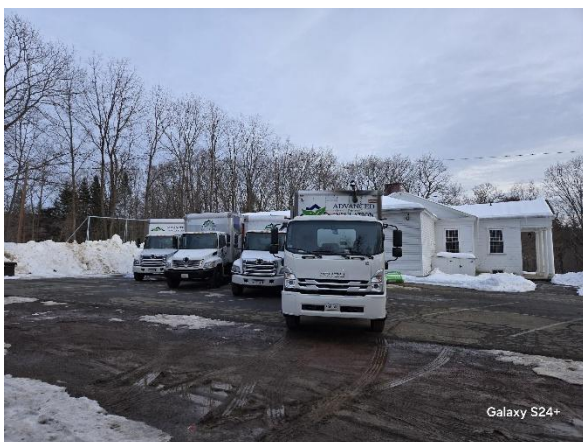
Insulation workers at the Fellowship Hall
